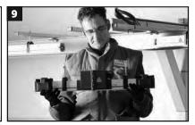
The electrical supply can be made either at one end of the line, end supply (Photo 8) Or it can be made by connecting at any of the section joints along the installation, intermediate supply (Photo 9).
