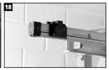
Install the corresponding towing arm RGMM06 or RGMM08, aligning it with the central axis of the conductor bars, and slightly lower than the collector trolley. It is very important that the pulling is parallel to the axis of the line. The collector trolley cable should be installed forming sufficient loop, to not cause any torsion of the trolley (Photos 19 and 20).
