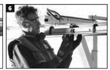
Cover the connection, sliding the **joints RGMM02** (**both halves**) (Photo 6) until completely closed (**click**) using the pressure tabs (Photo 7).
